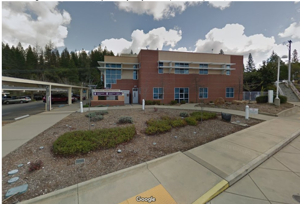
Figure 2: Marshall Way view of Project Site (Source: Google 2018)
